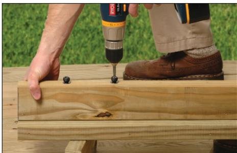
**Step 2:** Fasten FastBall™ connectors on each mark using the screws provided. Use the circle washer when using treated lumber to prevent direct contact. Simply place the washer in between the rail and FastBall connector.
