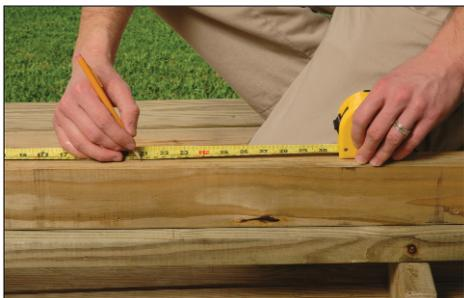
**Step 1:** Mark top and bottom rails 4-1/2" on-center starting from the center of the rail.
