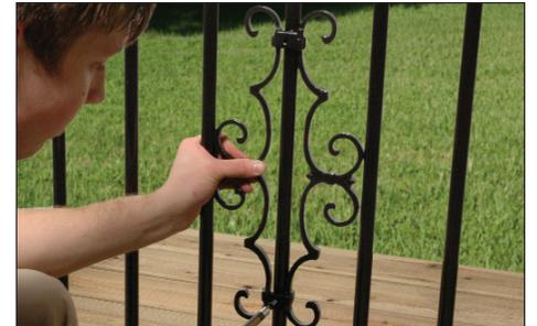
**Step 8:** If applicable, attach centerpiece to center baluster using the screws provided. Turn centerpiece so screws face out.
