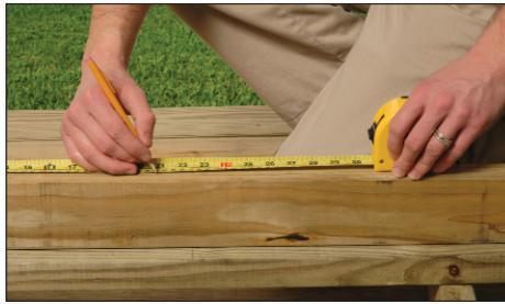
**Step 5:** Measure and mark top and bottom stair rails 5-1/2" on-center starting from the center of the rail.
