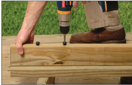
**Step 6:** Screw FastBall connectors on each mark using the screws provided. Use the oval washer when using treated lumber to prevent direct contact. Simply place the washer in between the rail and FastBall connector.
