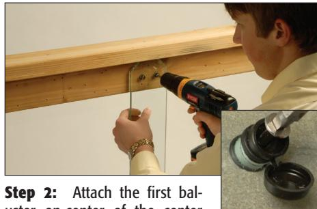
**Step 2:** Attach the first baluster on-center of the center line using four of the screws provided. Place screw cap in between rail and screw. Drive each screw until the rubber washer begins to mushroom. Do not over drive. Snap cap into place to conceal screw head.
