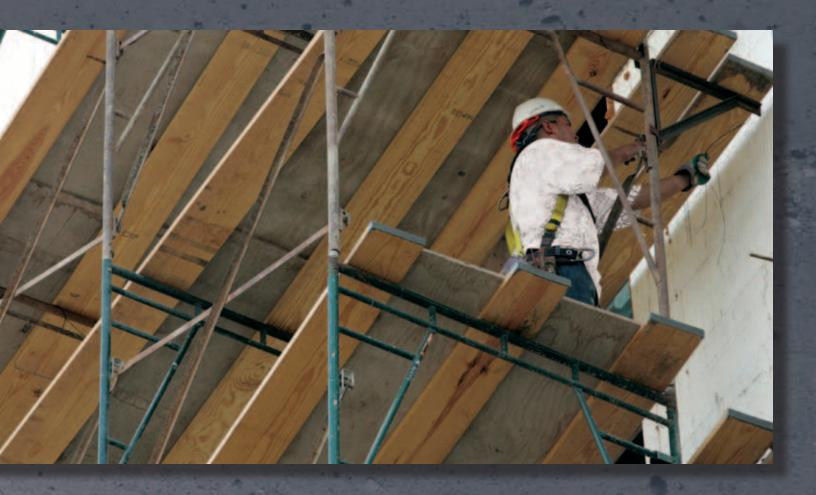
Scaffold planks take a beating, so Universal Concrete Forming Products OSHA-stamped scaffold planks are made of durable, engineered wood LVL or solid-sawn dimensional lumber. These scaffold planks can withstand rain, snow, heat, cold, heavy loads, and wear and tear from numerous assembly and knockdown cycles.
