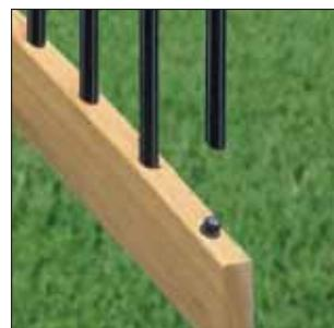
**Step 7:** Slide the trimmed balusters over each FastBall baluster connector on the bottom rail. Use a rubber mallet to tap the balusters onto the connectors if needed. Install the top rail, fitting balusters on each FastBall connector as you work across. Gently tap the top rail with a rubber mallet to eliminate any gaps. Secure handrail to post according to local building codes.
