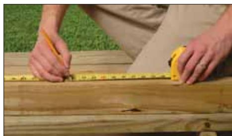
**Step 5:** Measure and mark top and bottom stair rails 5-1/2" on-center starting from the center of the rail.
