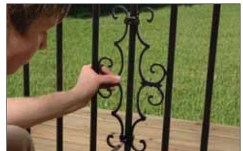
**Step 8:** If applicable, attach centerpiece to center baluster using the screws provided. Turn centerpiece so screws face out.
